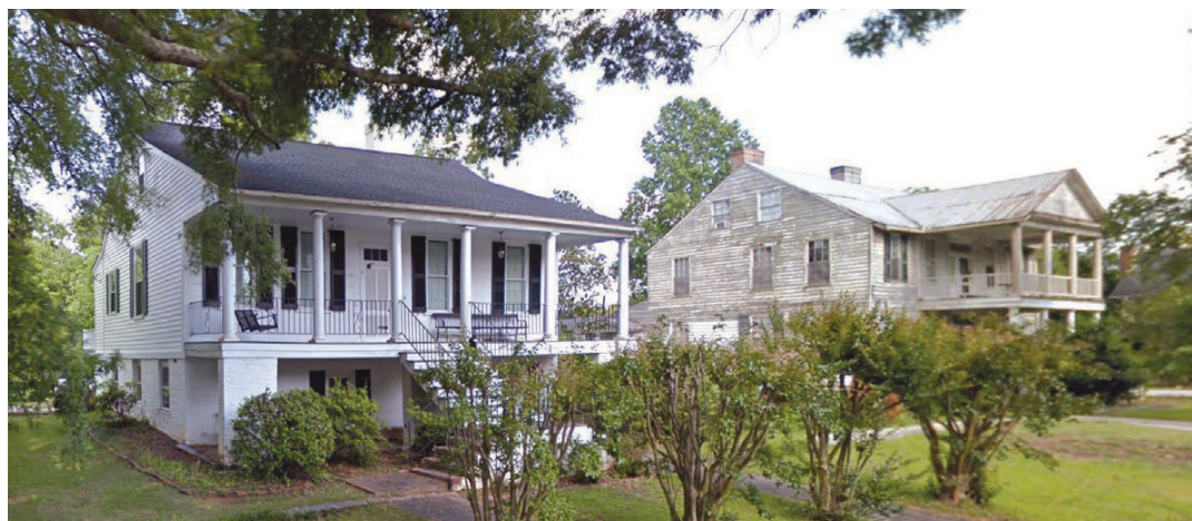
102 North Zion Street (9) and 100 North Zion Street (8)
