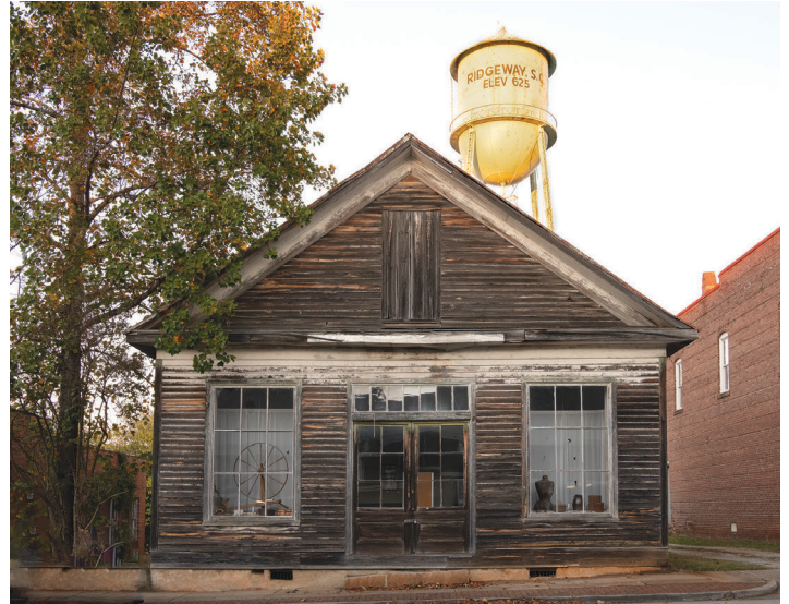
Ruff & Cloud Mercantile (11), Ridgeway Water Tower (12)
